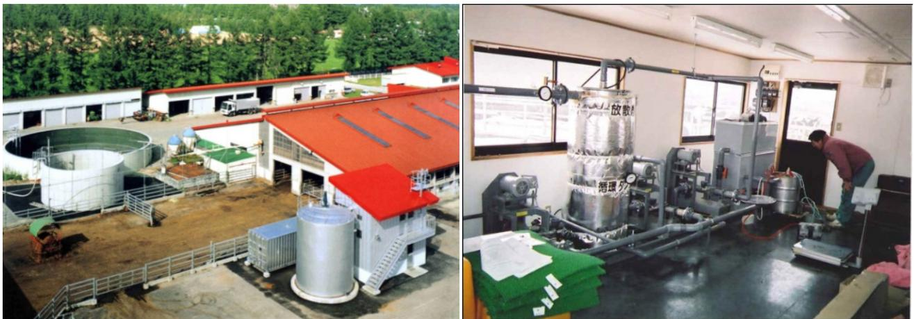
**Fig. 3** Thermophilic biogas plant (4 tons per a day) and bench scale ammonia stripping plant attached to the biogas plant in Obihiro University of Agriculture and Veterinary Medicine
